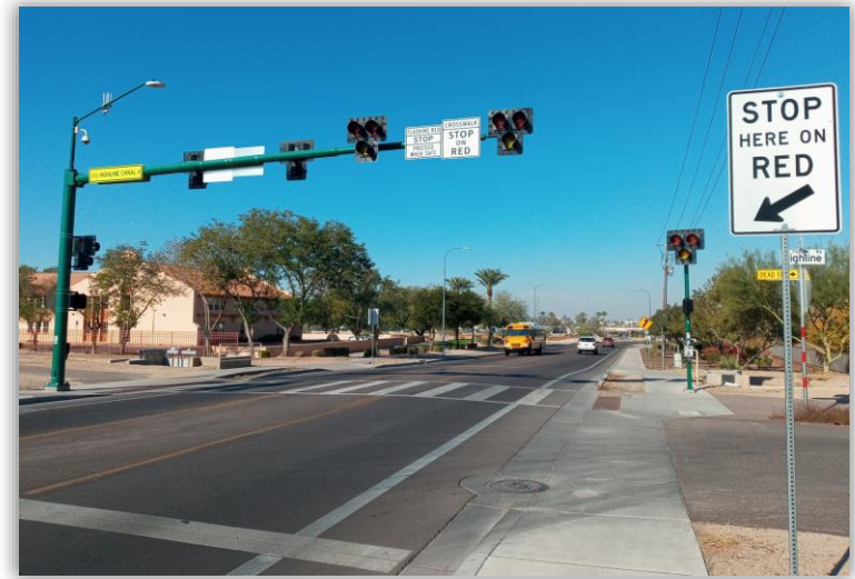
The Hawk Signal at 8025 South 7th Street (Highline Canal) was Activated in January
