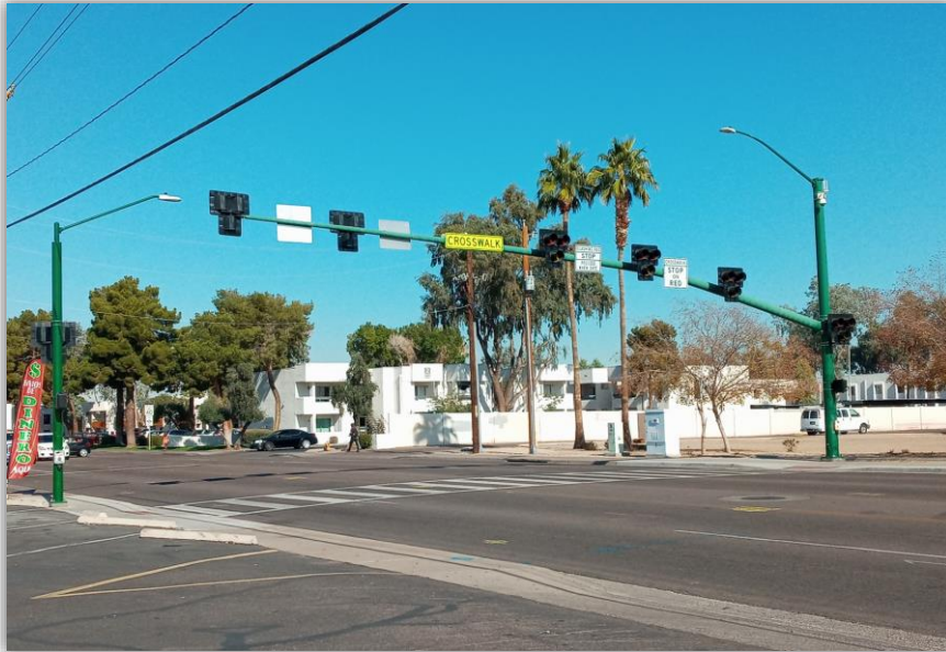
The Hawk Signal at 6104 N 27 th Avenue was Activated in December
