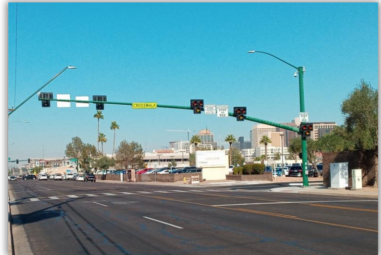
The Hawk Signal at 1215 South 7th Avenue was Activated in October
